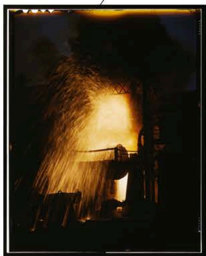
Bessemer converter (iron into steel), Allegheny Ludlum Steel[e] Corp., Brackenridge, Pa.
